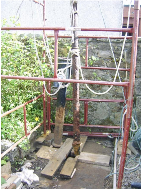
The down pipe is an 8ft long cast iron pipe some 3½" OD and 2¾" ID with a 7" dia joining flange. I don't know its exact weight, but I can only just lift it.
